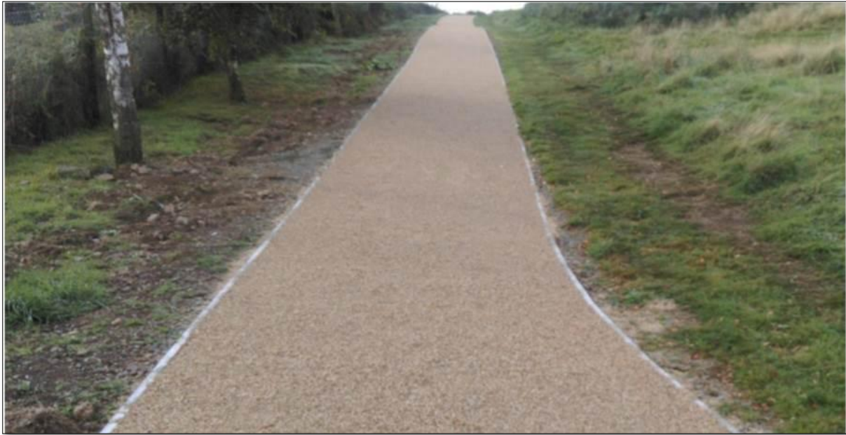
Figure 23 Typical Greenway Construction
